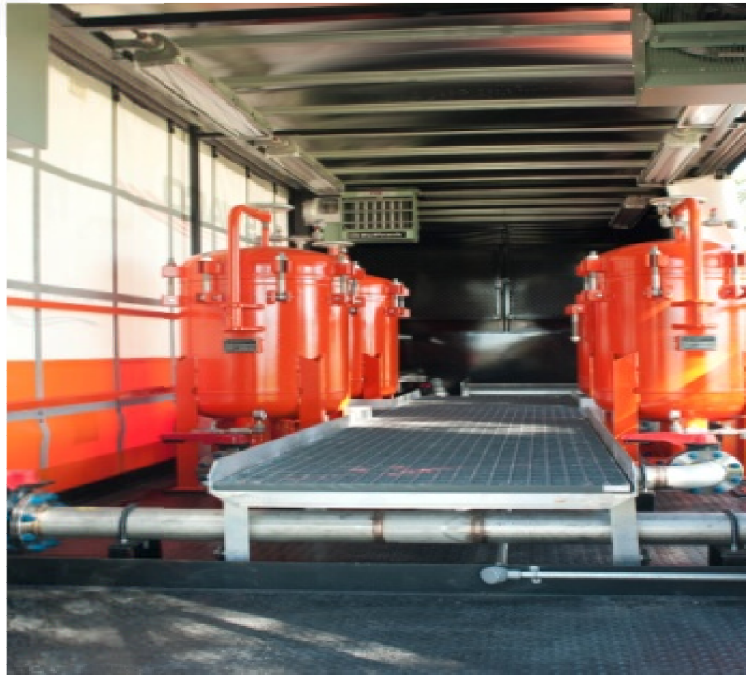
Figure 4.3 Filtration pods.
