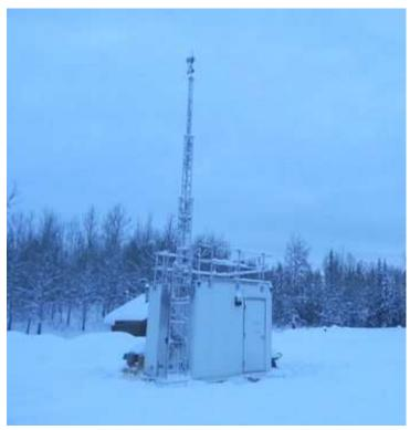
Figure 2 The new air quality station at Doig River. All three of the new air quality stations were installed in December 2013 and monitor sulphur dioxide (SO2), total reduced sulphur (TRS) and meteorology including air temperature, relative humidity and wind speed and direction).
