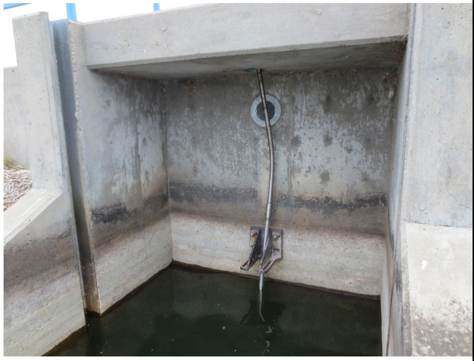
Gate Valve Stem Damage
