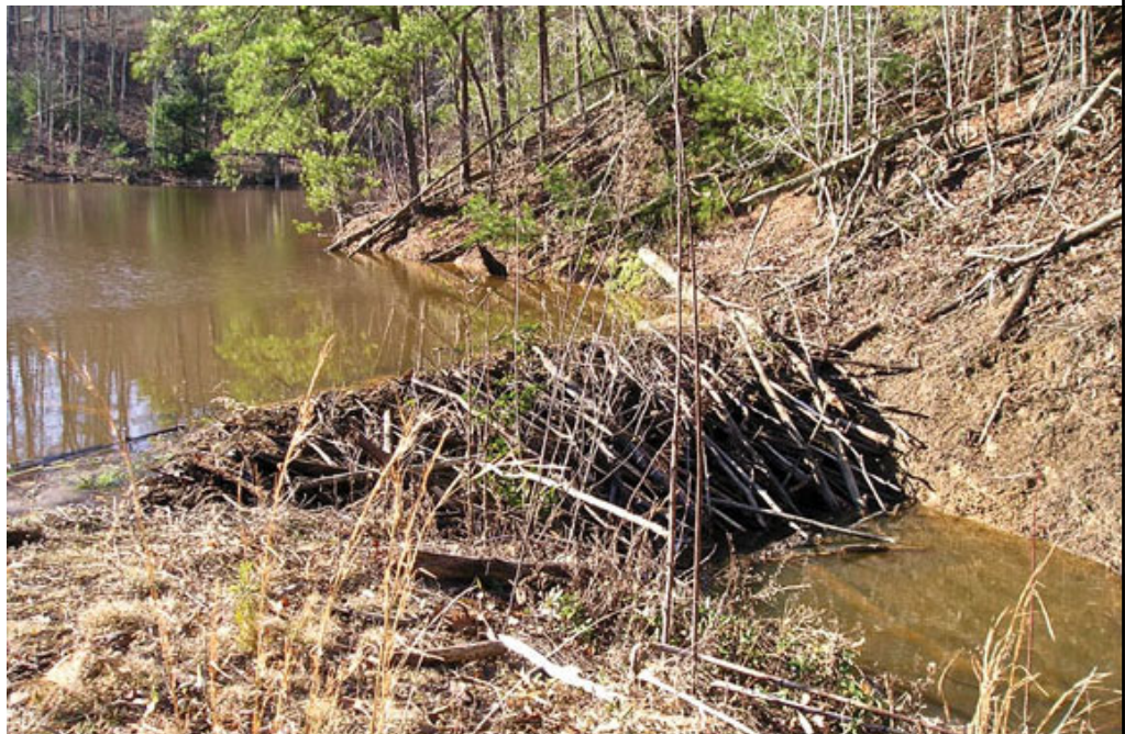
Blocked Spillway
