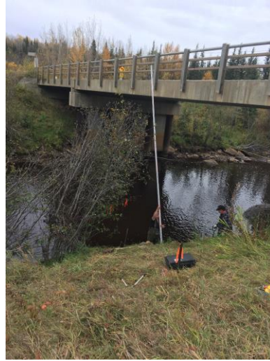
b. Surveying water level
