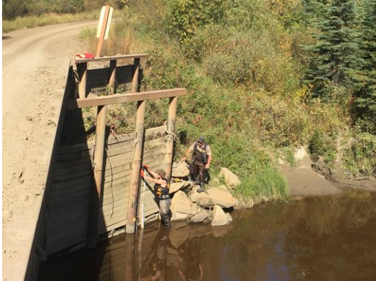
a. Installing staff gauge and logger.
