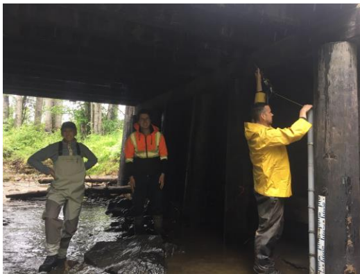
a. Re-installing equipment
