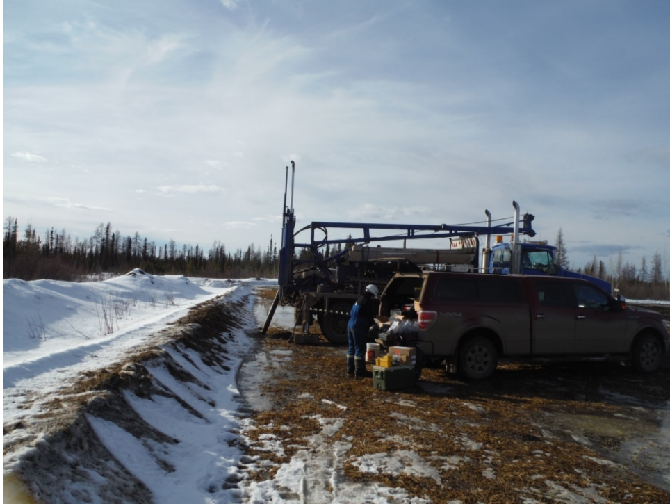
PHOTO 1: View of drill rig during collection of muskeg samples.
