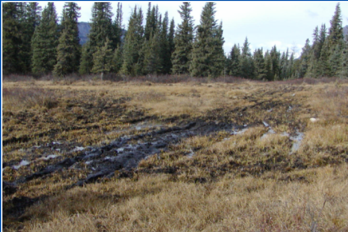
Example of water channelling down road which is used as access for recreational users. Road runs through fen resulting in drainage issues.
