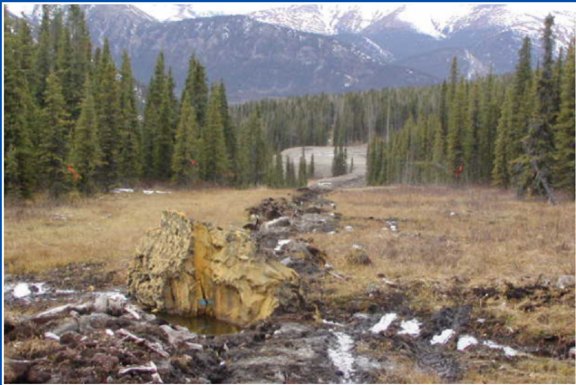
Ponding along access/pipeline due to poor drainage control. Foam berm used for drainage control ineffective and not properly installed.
