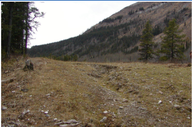
Erosion on slope down centre of access road.
