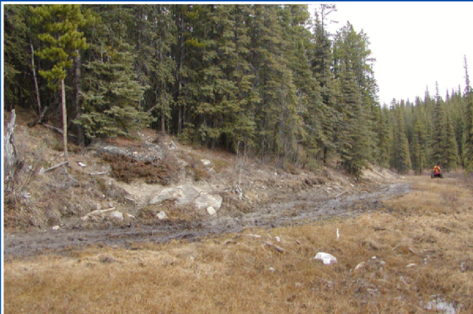
Seepage from upslope onto access road.
