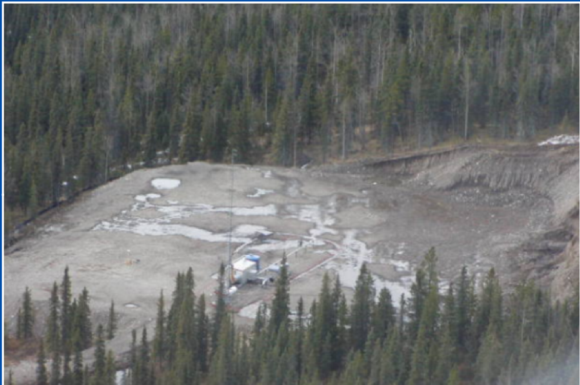
Upper slope failure, in spite of cutoff ditch being present. This suggests slope failure not due to surface runoff. Slope failure likely due to permeable soils and groundwater seepage.
