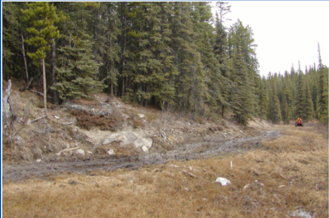
Example of road route selection through wetland when adjacent drier upland area would result in less ground disturbance (particularly with regard to ATV use).
