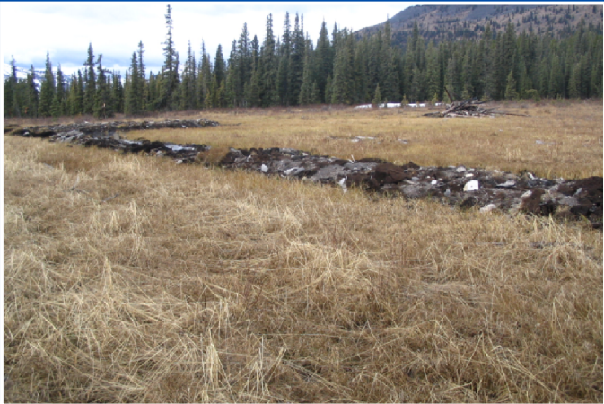
Pipeline trench within an open fen wetland.
