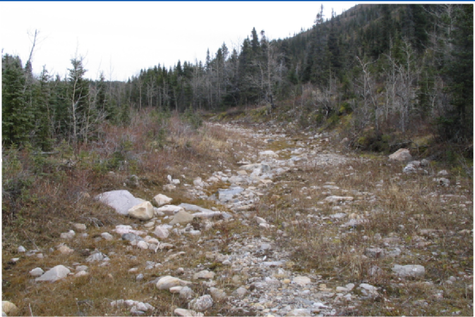
Erosion gully within access road down a slope, exposing rocks and cobbles.
