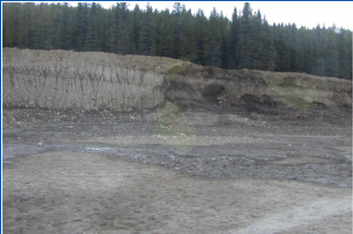
Well site showing cut and fill technique; including indication of groundwater seepage. Ungulate tracks present in wet areas.
