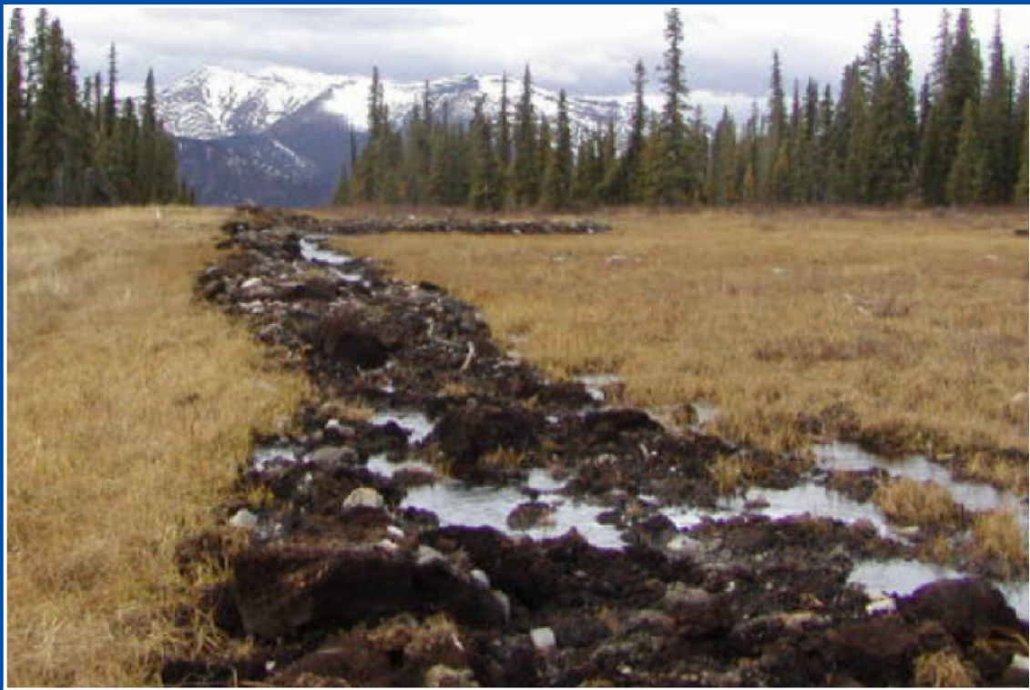
Installation of pipeline through fen without proper drainage management.
