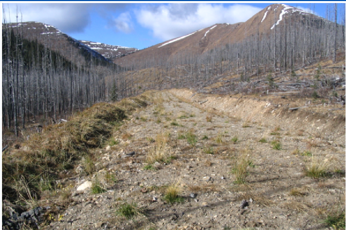
Removed surface duff layer along upland section of access road.
