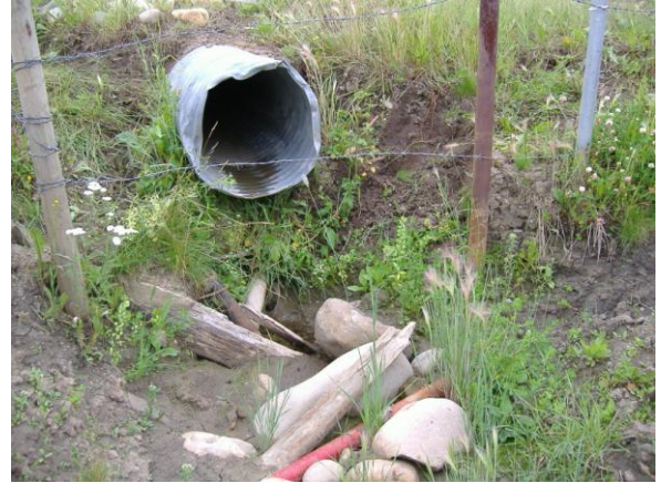
Figure 9 – Scouring and resulting gulying from perched culverts
