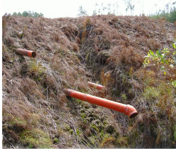
Figure 5 - Gully erosion from drainage pipe scour – 1.5m width (approx)
