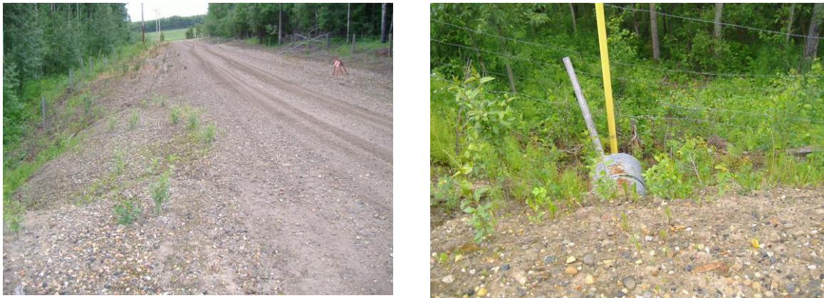
Figure 8 – Gullying, scouring and cracking on roadside near culverts
