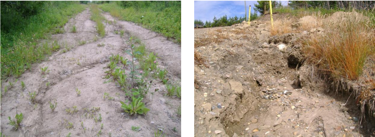
Figure 14 – Rilling and gullying on road surfaces and ditches, possibly benefit from waterbars
