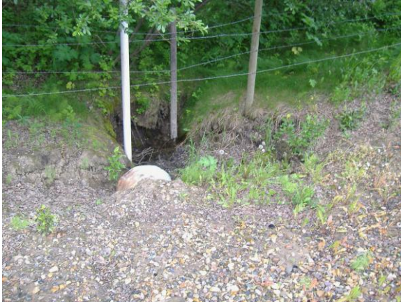
Figure 9 – Scouring and resulting gulying from perched culverts
