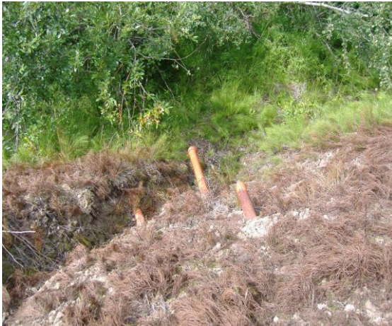
Figure 5 - Gully erosion from drainage pipe scour – 1.5m width (approx)
