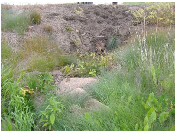
Figure 6 - Riprap placed in drainage pathway to mitigate scouring caused by dyke drain
