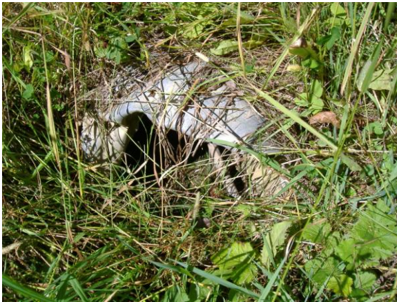
Figure 10 – Crushed and broken culverts
