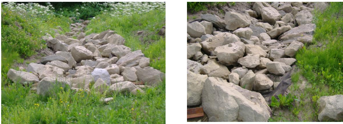
Figure 7 – Successful use of riprap and geotextile fabric at dyke drain outflow.
