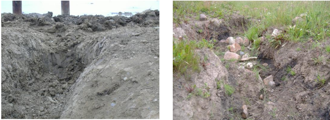
Figure 11 – Gullies around lease and in roadside ditch exacerbated by cattle access
