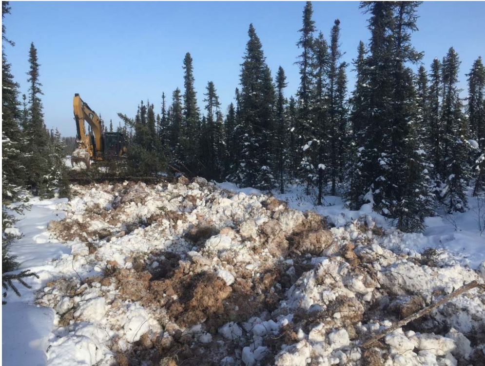
Photo 9: Tree-felling and Scarification by Ripping
