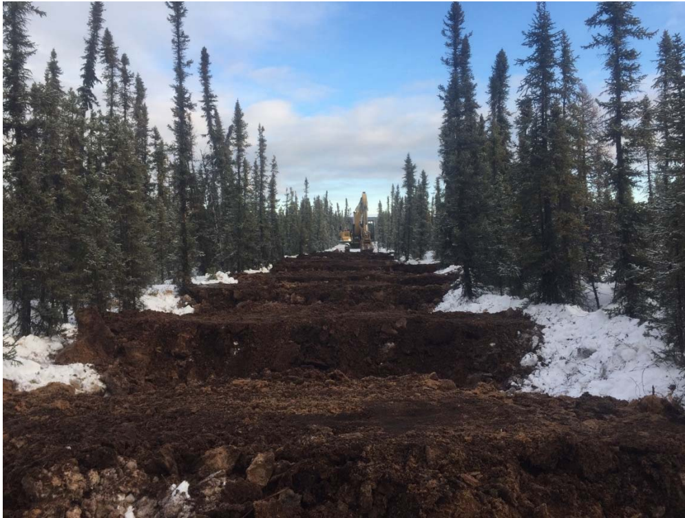
Photo 3: Mounding Using a Berm and Trench Style
