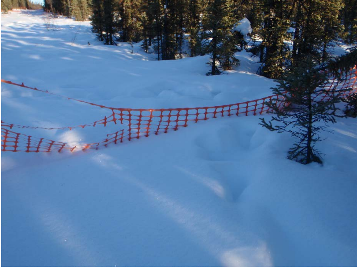
Figure A.2: An installed fence in winter: broken and crossed by tracks.
