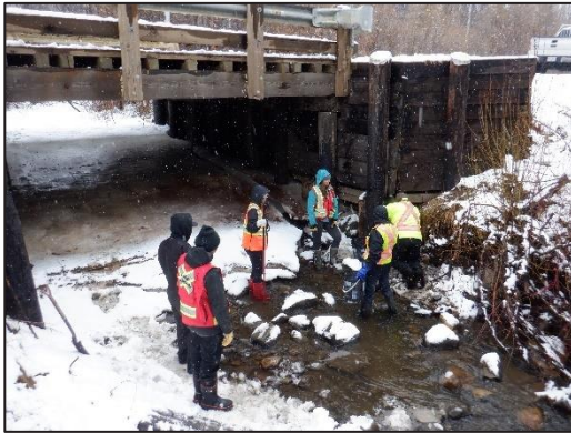
a. Reinstall equipment for spring melt. April 20, 2023.
