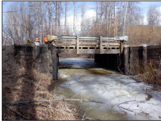
a. Reinstall equipment for spring melt. April 5, 2022.
