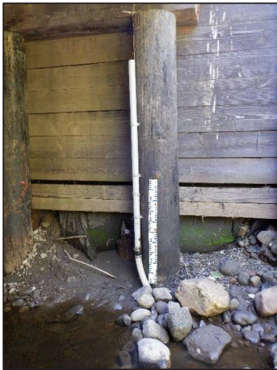
c. Armoring installation during low flows, July 27, 2022.
