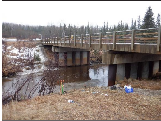
a. Reinstalling equipment for spring melt. April 8, 2022
