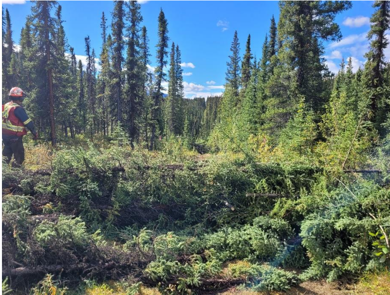
Figure 5: Trees dropped in a pile across the seismic line that was unsatisfactory as it was easy to climb over and unlikely to prevent the movement of animals down the line.
