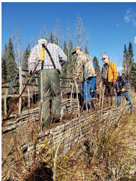
Building the wattle fence
