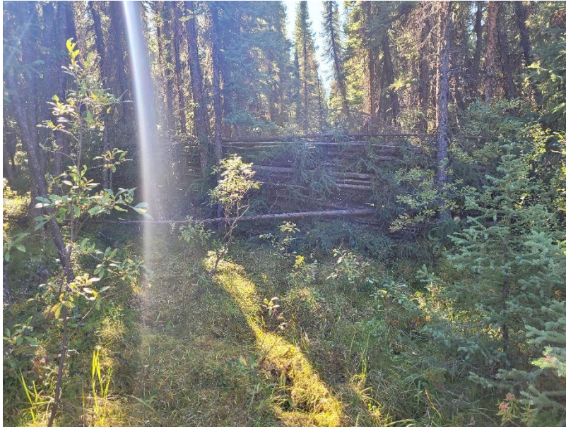
Figure 7: The completed brush fence spanned the width of the line, was densely built and hard to see through, and was installed using trees on either side to aid stability.
