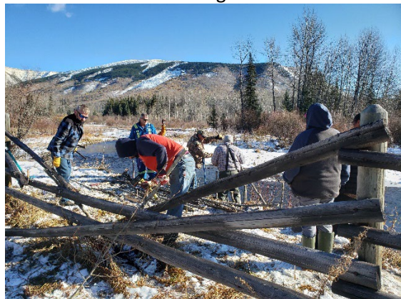
Wattle fence preparation
