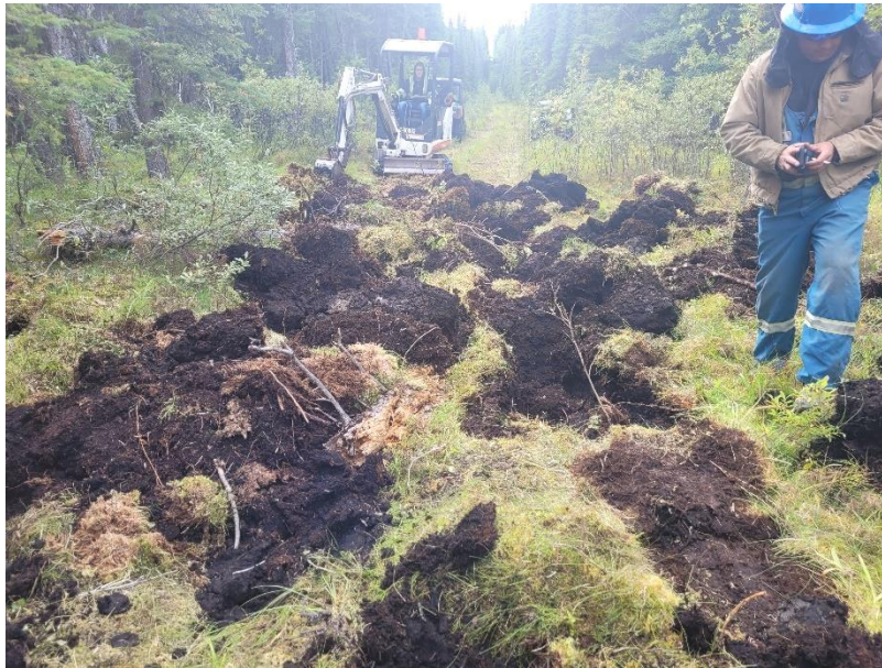
Figure 2: The operator practicing different techniques to dig the appropriate size and number of pits and mounds using the smaller machine.
