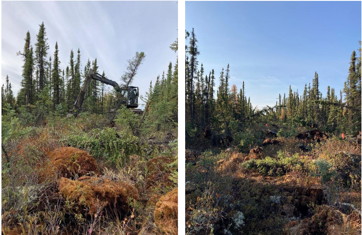
Figure 36. Close up of transplanted hummocks and tipped trees on a restored segment of line and flagged monitoring plots for follow-up visits in summer of 2023.
