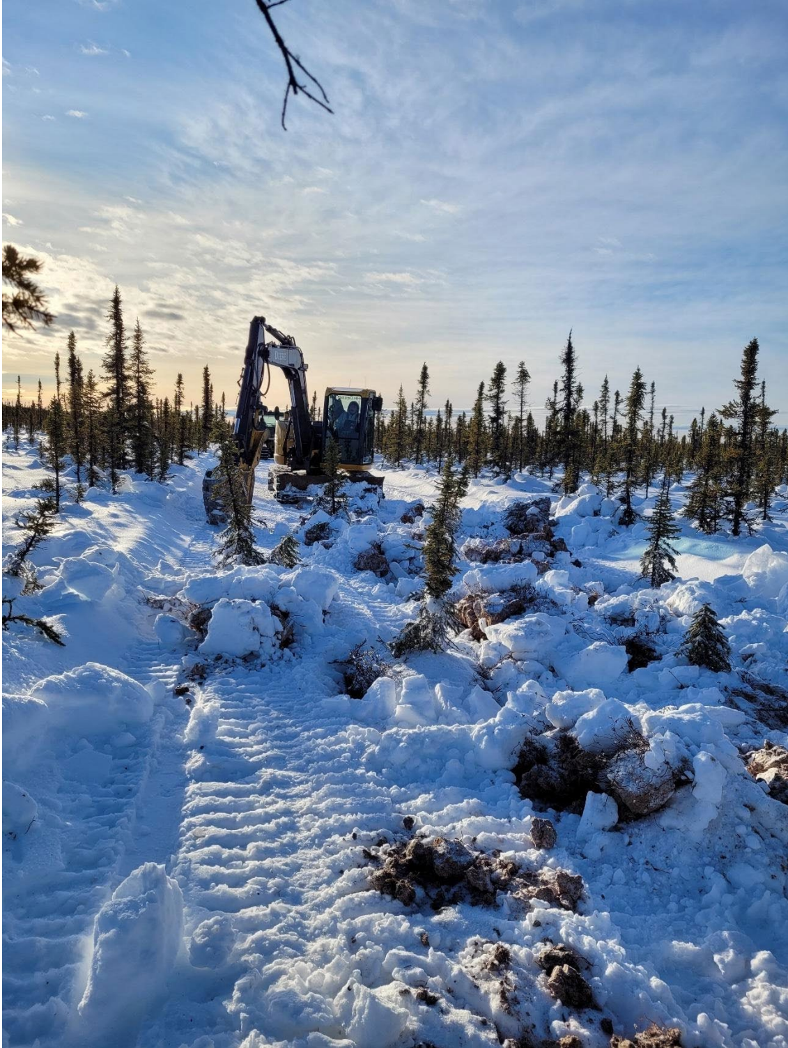
Figure 23. Implemented treatments during winter restoration in 2021-2022 in the Medzih'tene Restoration Area. Target lines were treated by transplanting hummocks and live black spruce trees from adjacent lines and by tipping liver trees over lines.
