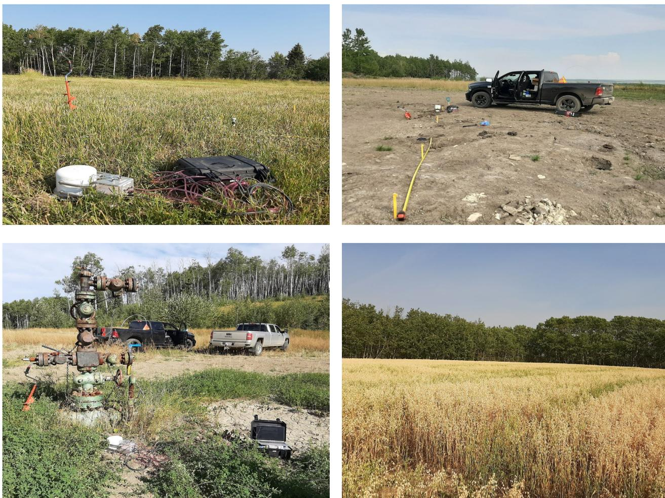
**Figure 6:** Varying conditions encountered at investigated P&A well sites showing; a cut capped and buried well, with reclaimed vegetation in a grazing field (top left), a very recently reclaimed site with no vegetation growth and presence of “pock marks” and bull dozer tracks (top right), a disconnected well head and valve assembly (bottom left) and a fully reclaimed crop field (bottom right).
